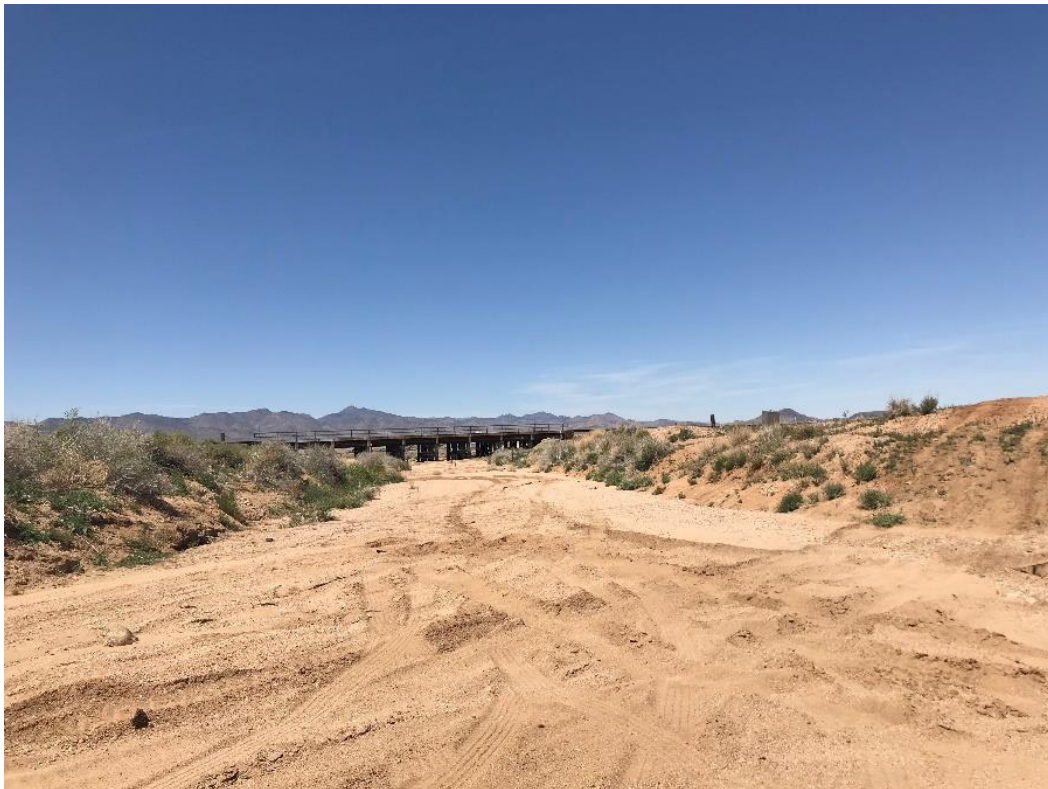
Photograph 6. View looking north from Industrial Boulevard towards BNSF railroad bridge over Rattlesnake Hill Wash.
